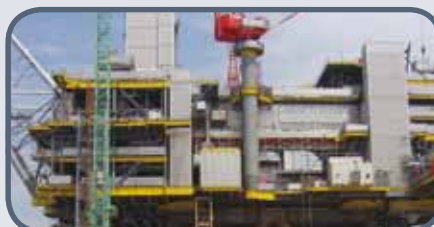
Gas & Oil Facilities
